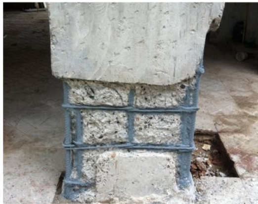
TYPICAL IMAGE OF SURFACE PREPARED RCC MEMBER
