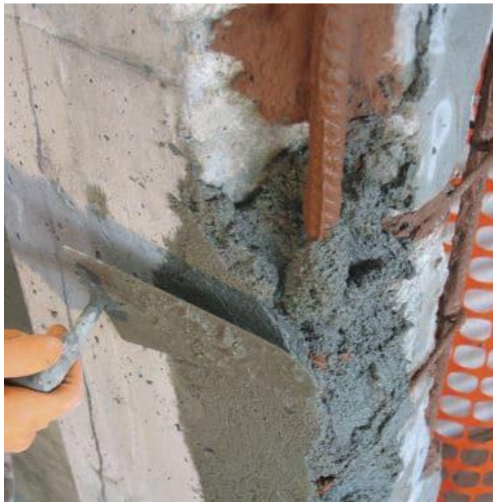
Fig. 3: Polymer Modified Mortar Used for Restoration of Piles
