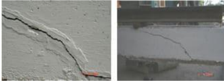
Fig. 2: Repair Cracks in Reinforced Concrete Beams using Polymer Modified Mortar
