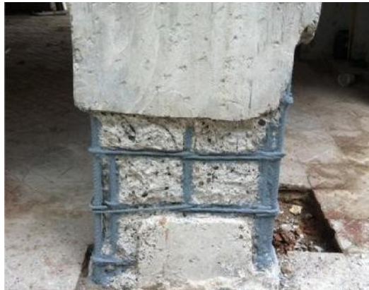
TYPICAL IMAGE OF SURFACE PREPARED RCC MEMBER
