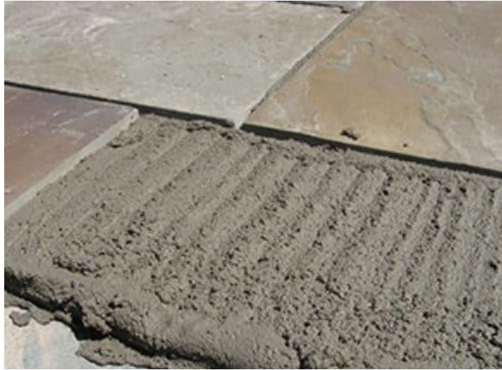
Fig. 4: Use of Polymer Modified Mortar for Installing Tiles
